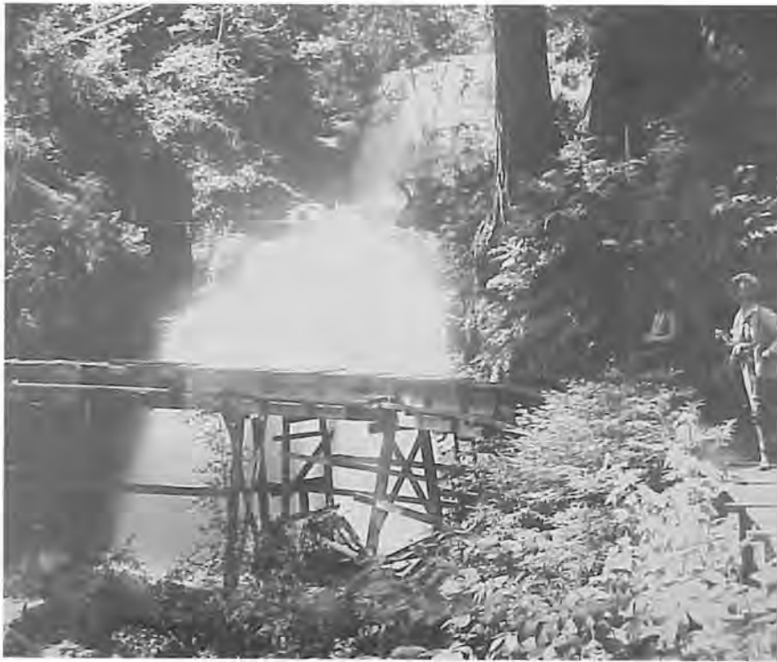
An eighteen-mile flume was constructed to carry logs south from Waterman Gap to the town of Felton.
